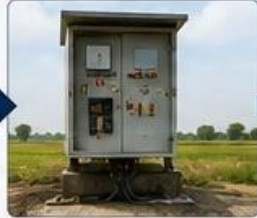
SOLAR CONTROLLER INSTALLATION
