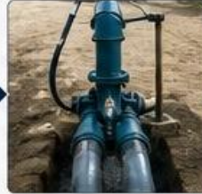
SOLAR PUMP INSTALLATION
