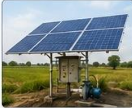
SOLAR STRUCTURE INSTALLATION
